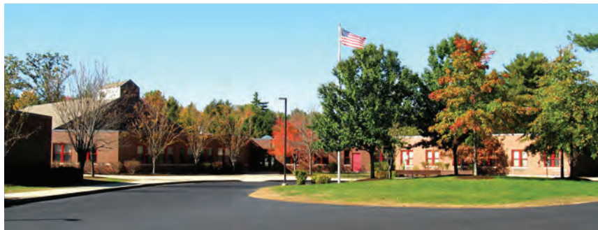
Acton Elementary School in Acton, Maine.
